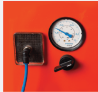
Vacuum gauge provided to check the leakage of the valve seat
